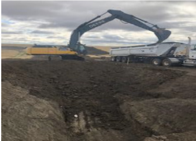
Loading trailer with contaminated soil – Sept 27, 2018
