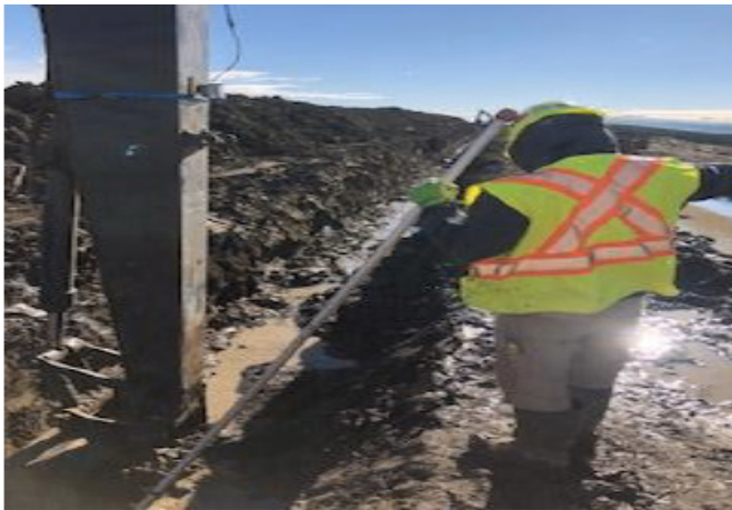
Excavator and swamper shading pipe - km 145+150 – Sept 28, 2018
