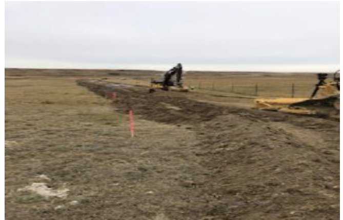
Excavator pulling dams out of watercourse – SF 97 –Sept 26, 2018
