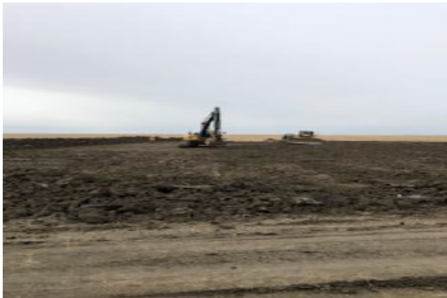
Access approach being constructed – SF 158 – Sept 26, 2018
