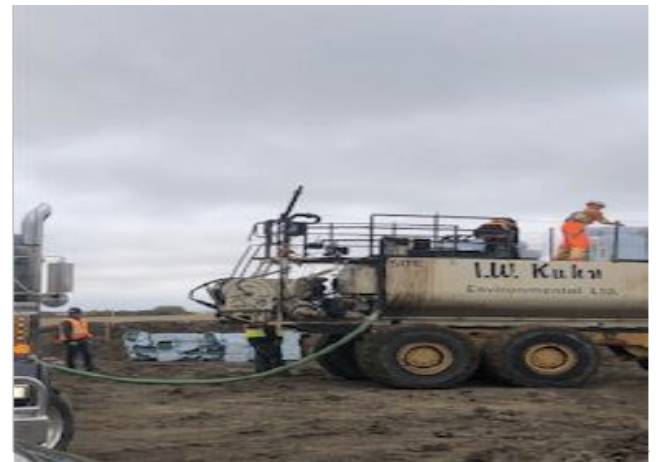
Crews unloading terra wood – km 145+950 – Sept 27, 2018
