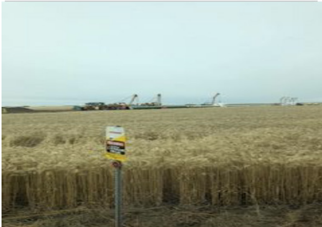
Mainline welding – SF 92 – Sept 26, 2018
