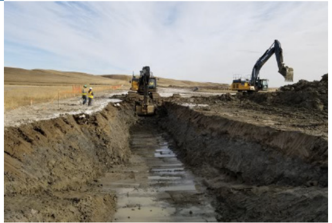
Digging bore pit on Heritage site – km 221+910 – Sept 28, 2018
