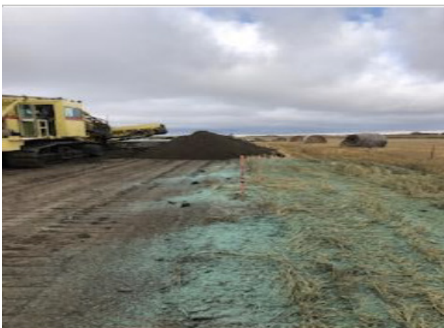
Terra wood sprayed at spill pile – Km144+900 – Sept 27, 2018
