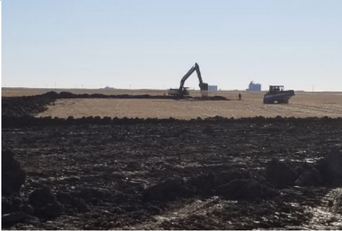
Equipment moving dirt – km 259+150 – Sept 28, 2018
