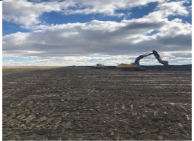
Topsoil being stripped – km 234+100 – Sept 27, 2018
